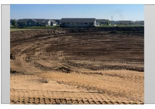
Baseball field topsoil stripped and read for fill
