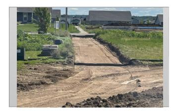
Sidewalk heading out to Porter Ave. cut to subgrade and compacted
