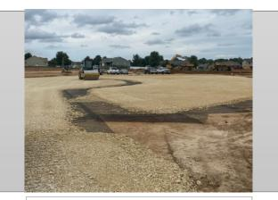
Parking lot 3" base stone being installed and compacted over geo-grid
